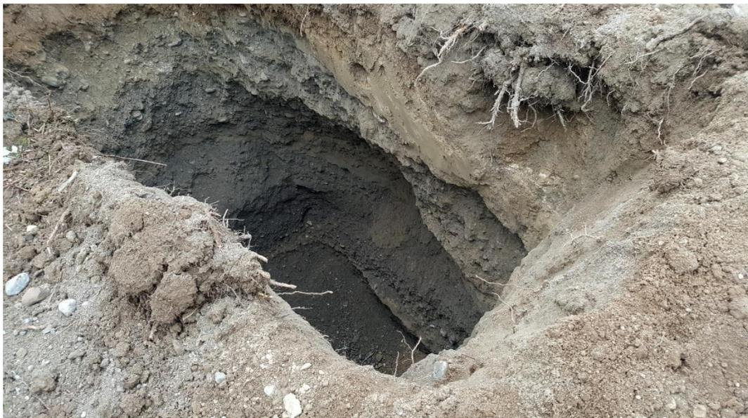
*Figure 6. Trial pit for bulk sample.*
